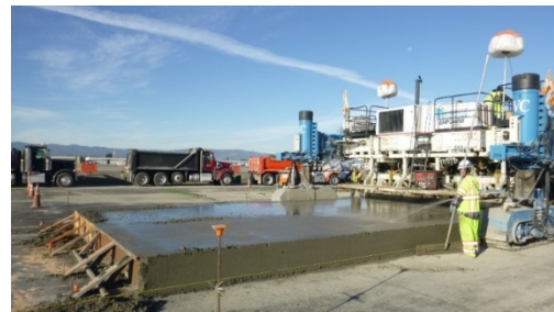
Terminal B Ramp Rehabilitation
