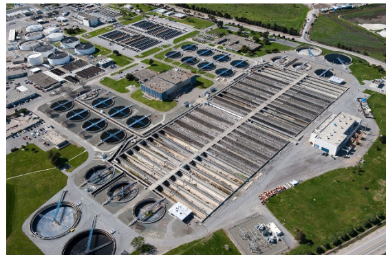
Aerial View of the San José-Santa Clara Regional Wastewater Facility
