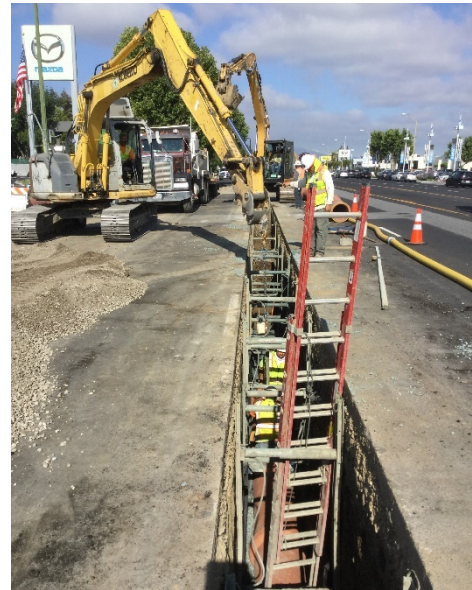
Stevens Creek Sanitary Sewer Replacement
