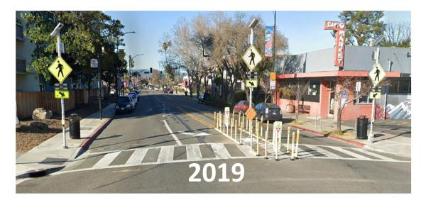
Rectangular Rapid Flashing Beacon installed in 2013 and upgraded in 2019
