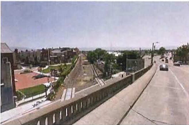
Looking West to Project Site from Overpass
