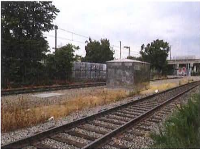
Looking Northeast to Project Site from Rail Tracks
