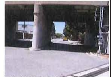
Looking North to Dupont Street Below Overpass
