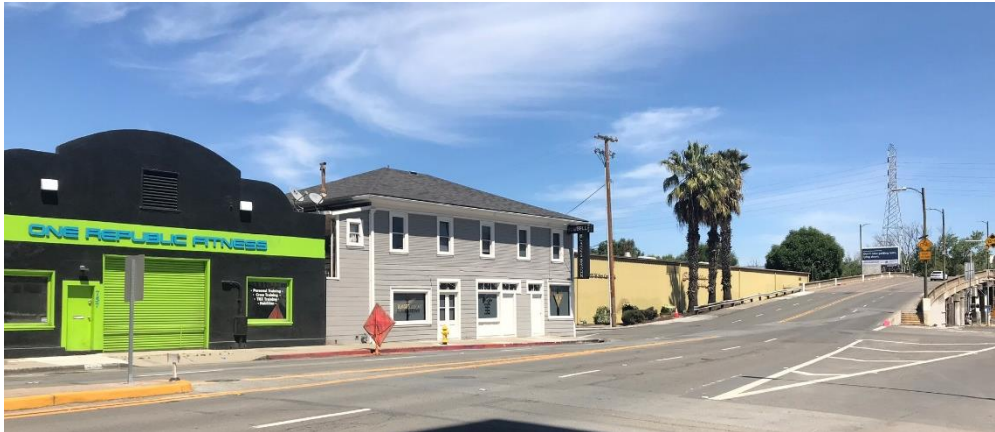
Figure 6: 751 W San Carlos (center) with 757 W San Carlos left of frame ( April 22, 2020, camera facing northeast ).
