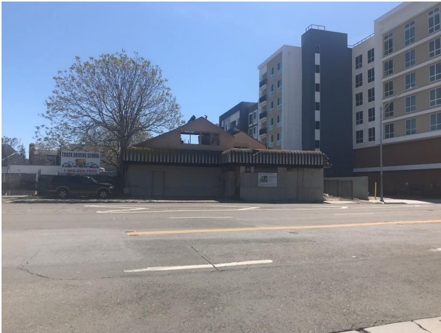
Photograph 6: North elevation, camera facing south, April 15, 2020.
