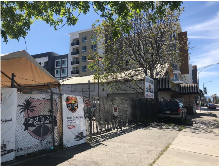
Photograph 5: North and east elevations, camera facing southwest, April 15, 2020.
