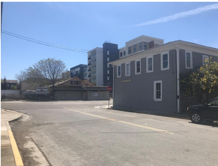
Photograph 7: North elevation of 750 W San Carlos Street seen from McEvoy Street, camera facing southwest, April 15, 2020.
