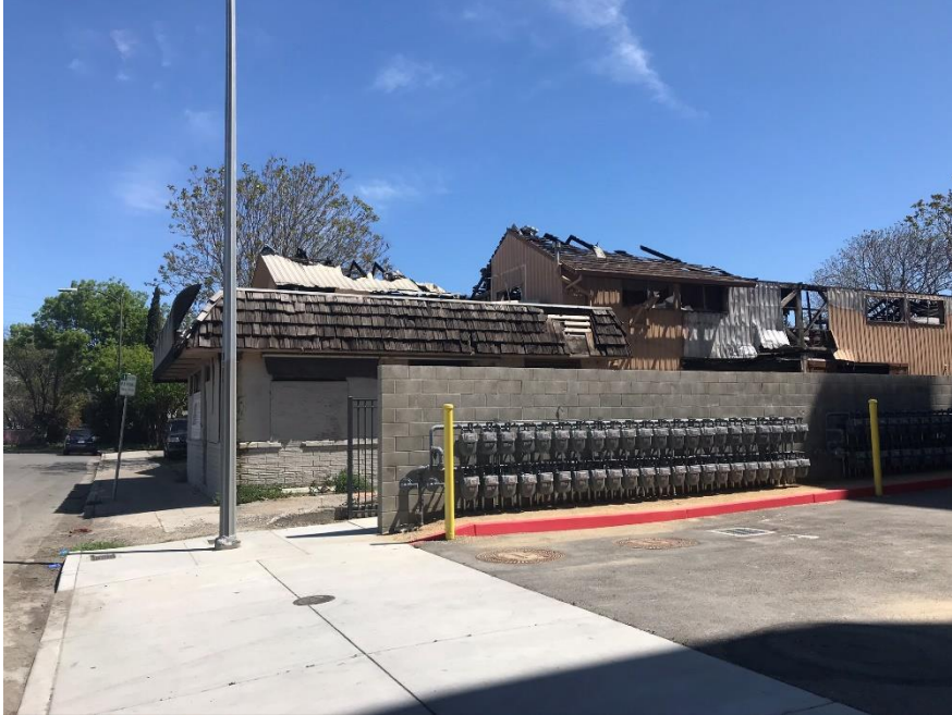
Photograph 2: West elevation, camera facing east, April 15, 2020.
