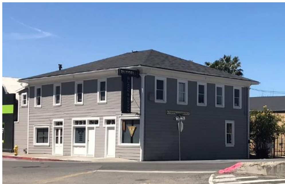
Figure 7: 751 W San Carlos ( April 22, 2020, camera facing northeast ).
