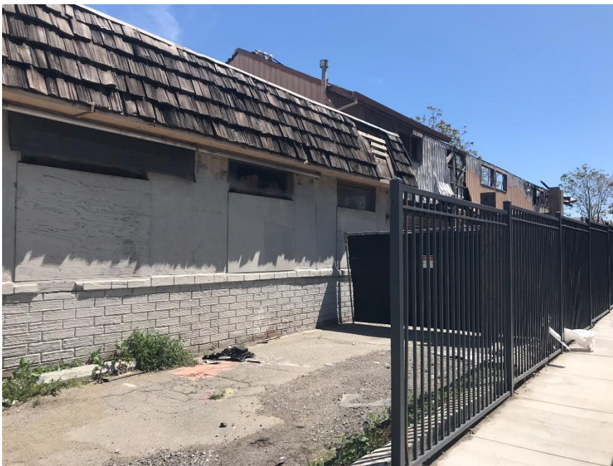
Photograph 3: Detail of front portion of west elevation, camera facing southeast, April 15, 2020.
