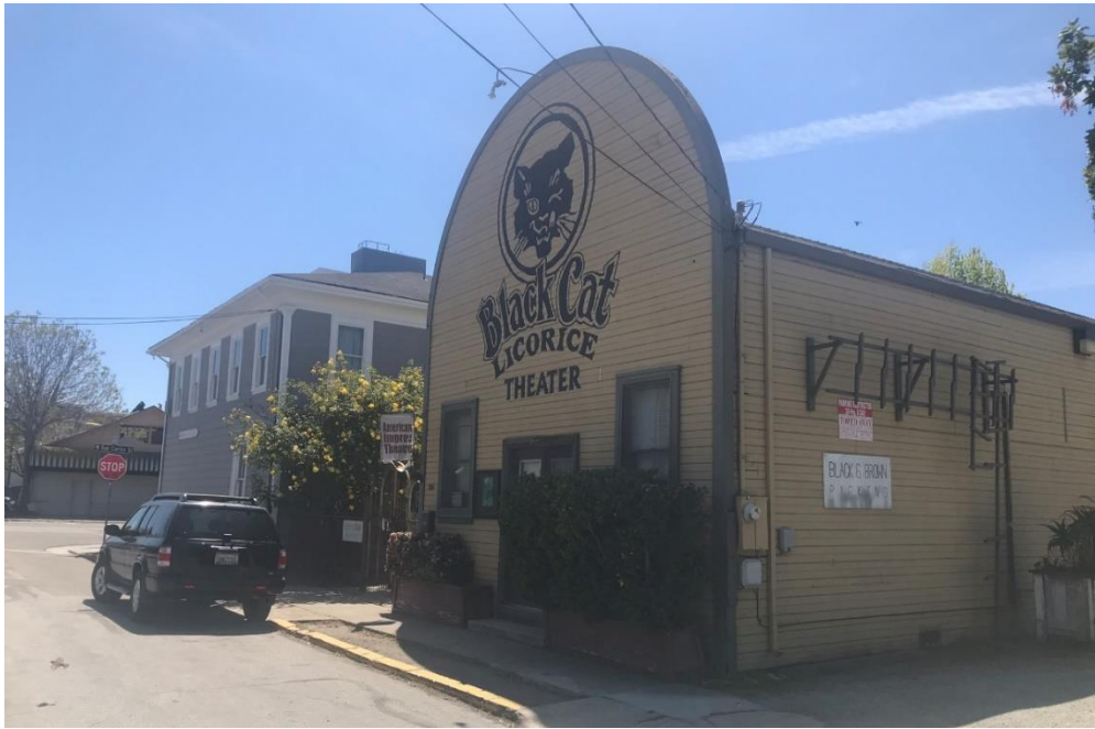
Figure 8:260 McEvoy Street with property left of frame (April 22, 2020, camera facing southwest).
