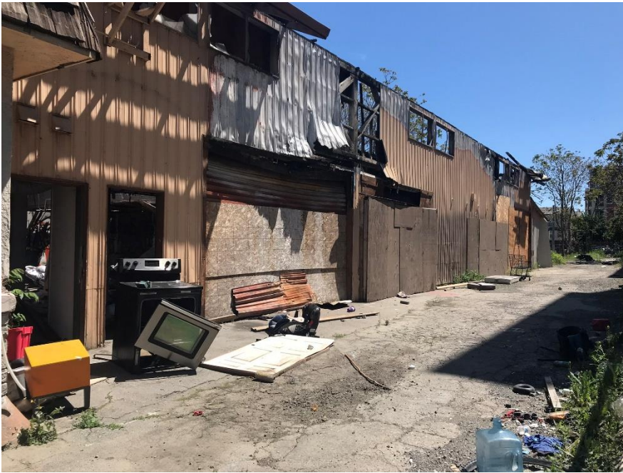
Photograph 4: Detail of back portion of west elevation, camera facing southeast, April 15, 2020.
