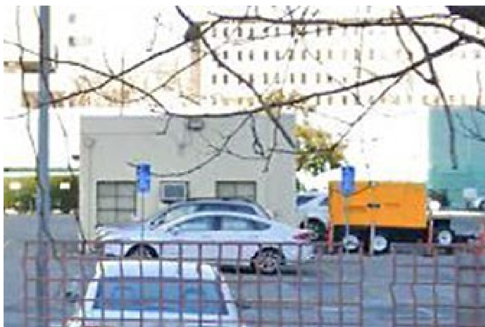
Photograph 3 Side facade facing Almaden Blvd.
