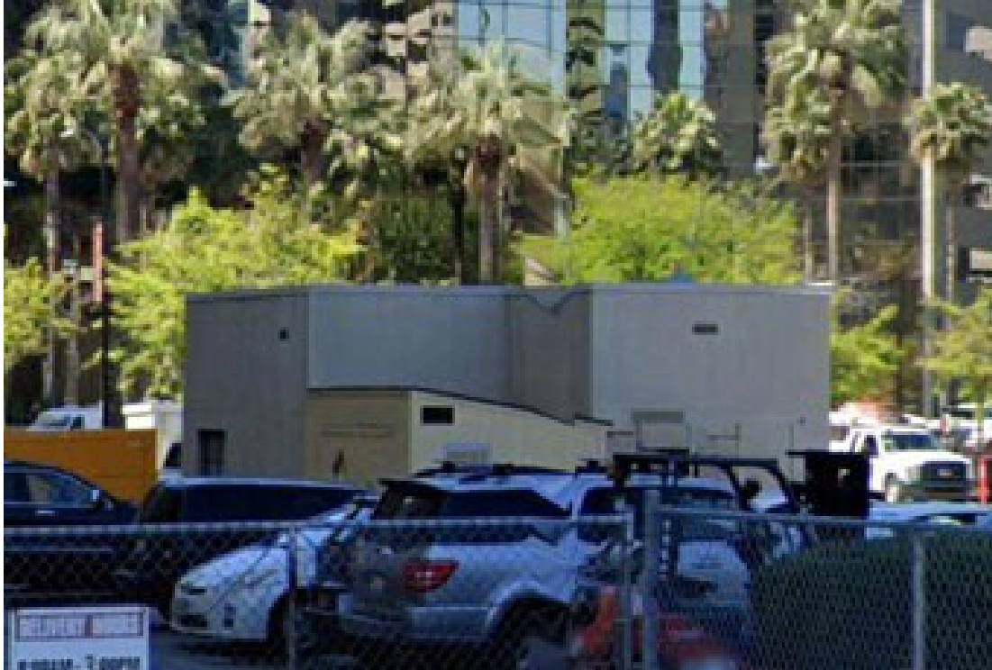
Photograph 4 Rear of the building showing the storage infill addition.
