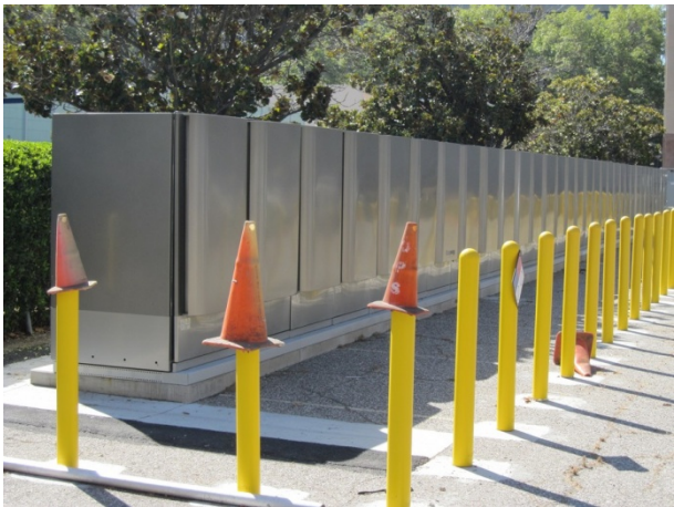
Photograph 5. Bloom Energy fuel cell installation.
