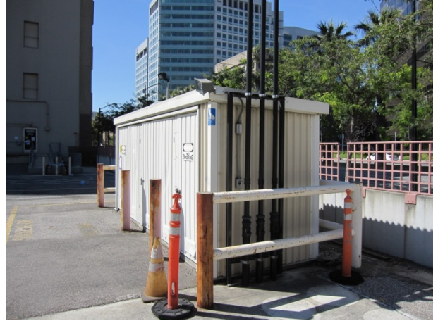
Photograph 8. Storage shed and UST vent pipes (former fuel pump house).
