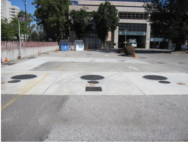
Photograph 7. Three diesel storage USTs.
