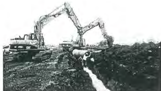
Taxiway W Phase IV Construction Underway
