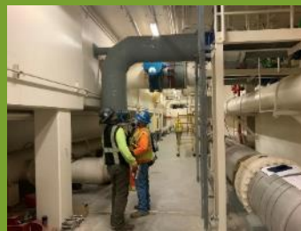
Contractors completing work in the nitrification tunnel.
