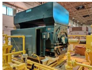
New electric motor installed on an existing blower
