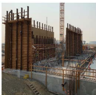
Installing vertical walls for the future grit basin building.
