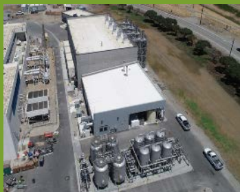
New Cogeneration Building 41.
