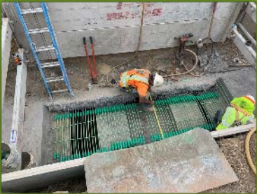
Contractors performing crown repair on a section of the 96-inch pipeline.
