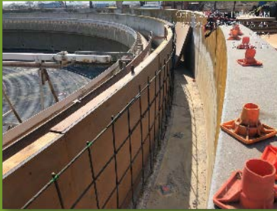
Rebar Assembly at Clarifier B2
