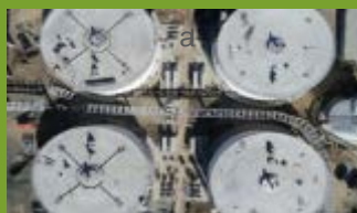
Aerial view of four anaerobic digesters at the RWF.
