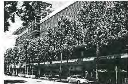
Fourth Street and San Fernando Parking Garage
