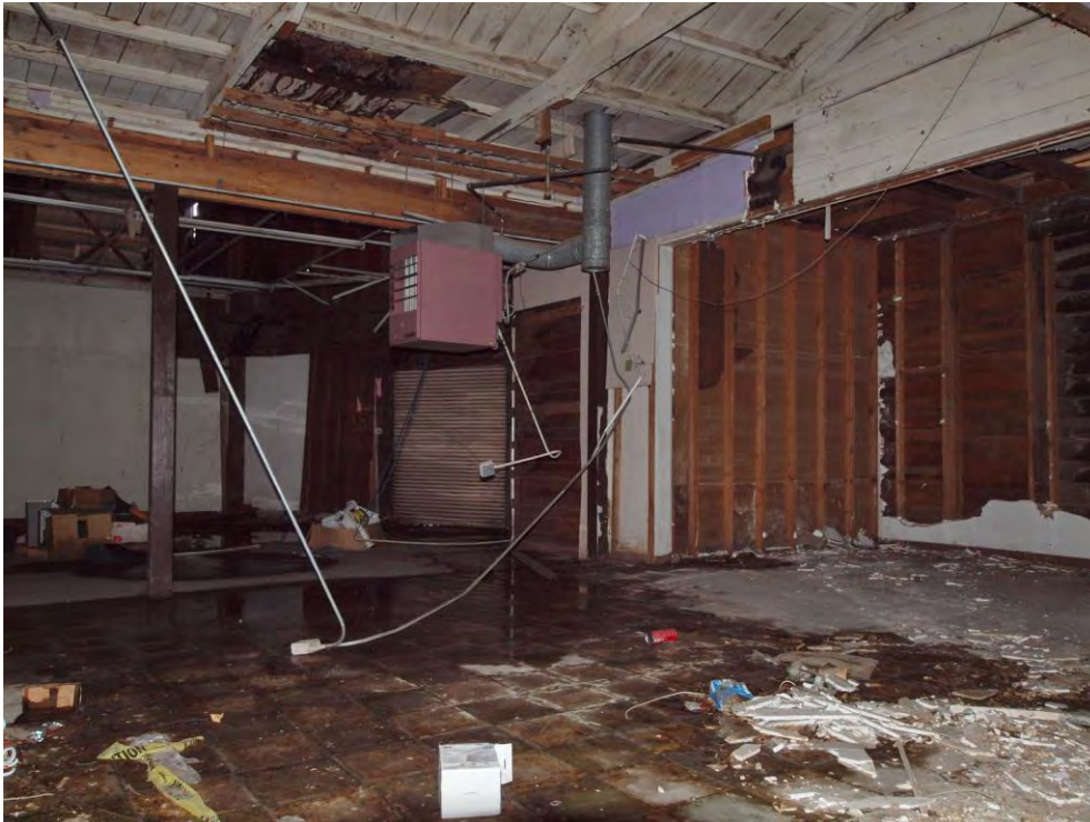
Rear addition area, viewed facing southeast.
