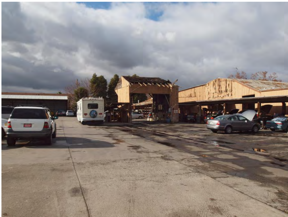
Rear of building, viewed facing west.
