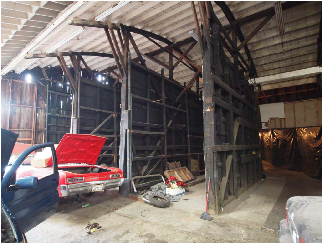
Original lumber store area, viewed facing southwest.
