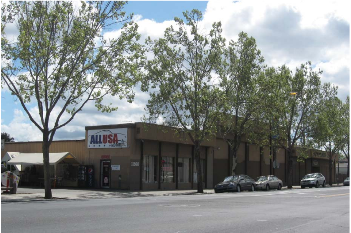
PHOTO 1: View of the project site, looking south from East Santa Clara Street.
