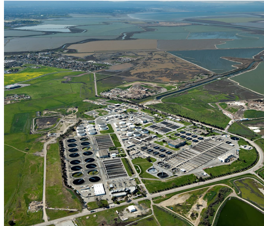
Aerial photo of the San José-Santa Clara Regional Wastewater Facility Source: Environmental Services Department
