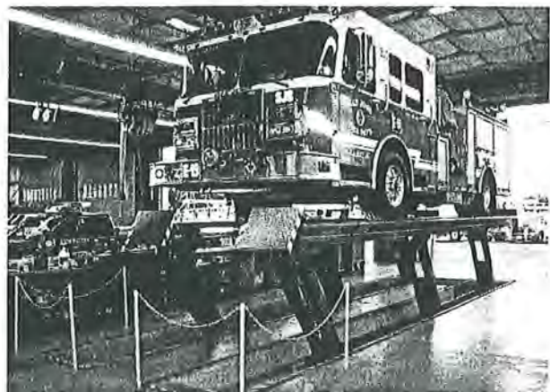
Fire Truck Maintenance at the Central Service Yard
