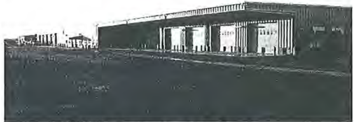
Central Service Yard Building F
