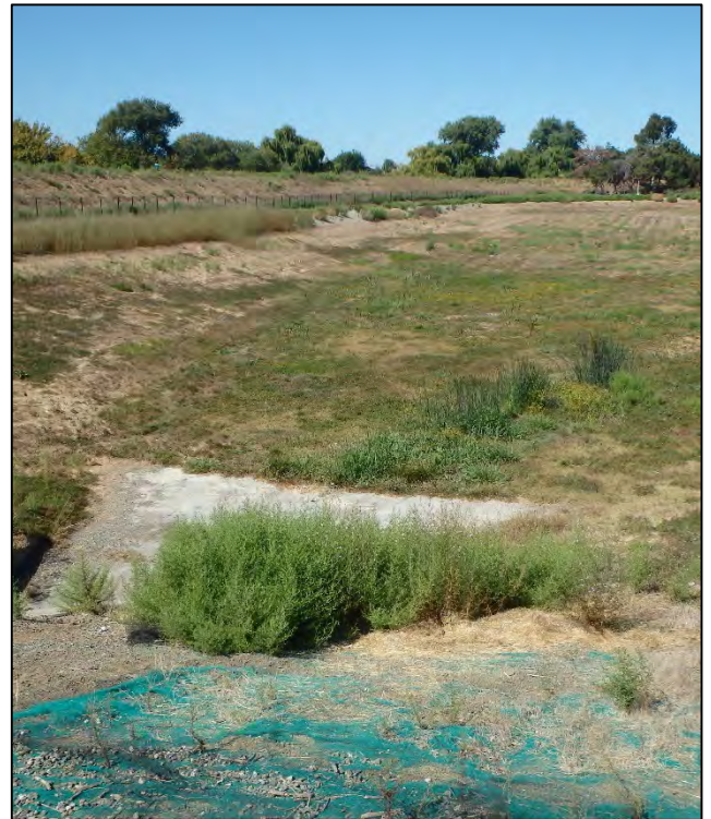
Photo 4. Looking southeast across the detention basin from the pump station.
