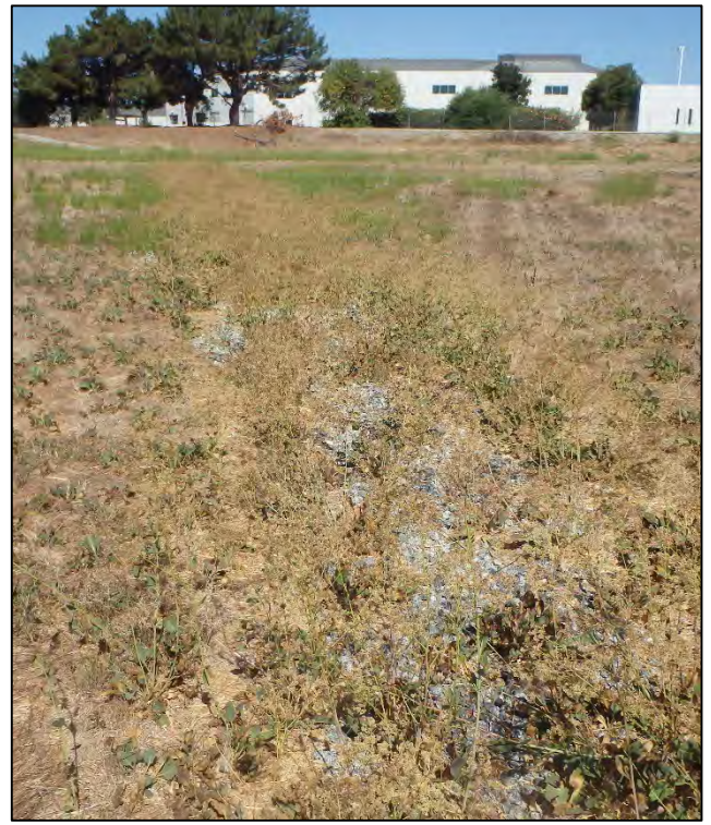
Photo 2. Looking north, showing the French drain in the middle of the basin.
