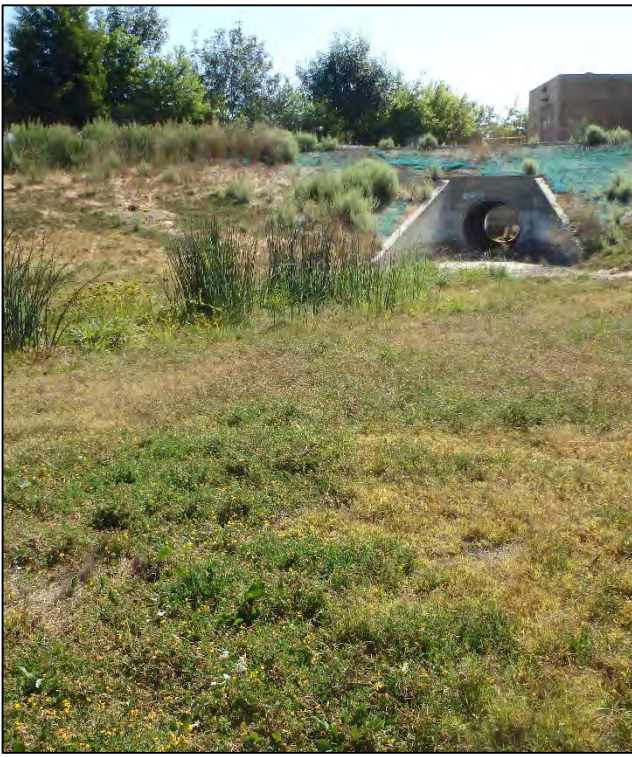
Photo 1. Photo showing small seasonal wetland located at pump station opening.
