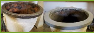
RAS elbow repairs: Before (left) and after (right).
