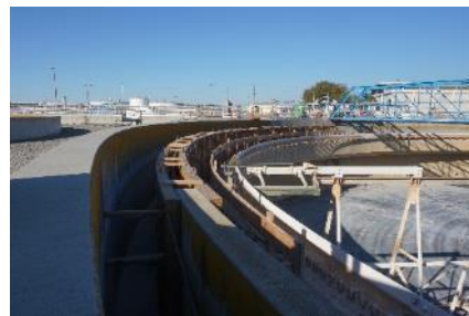
Nitrification clarifier wall rehabilitation
