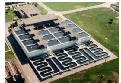
The RWF filtration system is critical to producing 99 percent-clean wastewater
