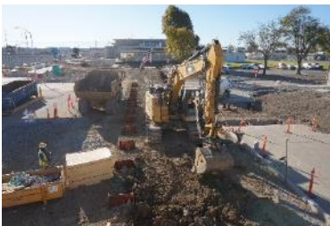
Excavation of the 96-inch pipeline trench for Headworks 3
