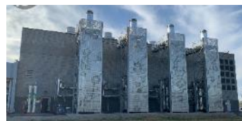
Cogeneration Building 41 engine exhausts with completed architectural facade.
