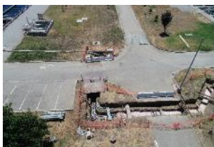
Electrical duct bank under construction.
