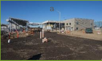
New Sludge Screening Building
