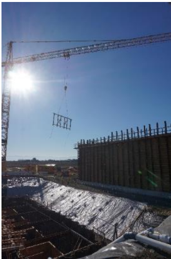
Construction on Grit Removal Facility at Headworks 3
