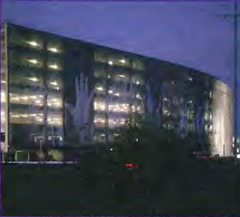
Airport Rental Car Garage
