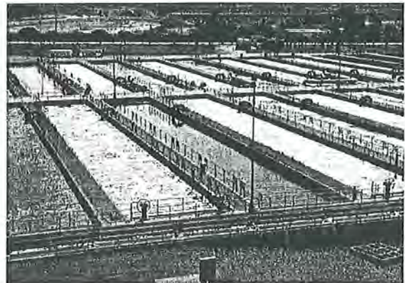
Secondary Aeration Tanks
