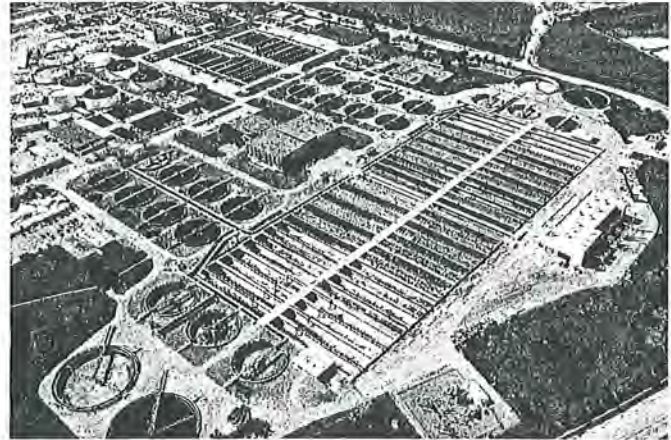
Water Pollution Control Plant
