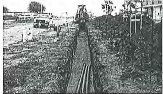
Fire Main Replacement - Phase 2
