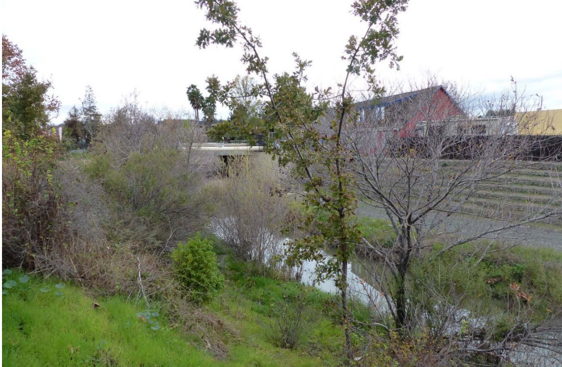
View of the bank of Lower Silver Creek from the property at 1948 Alum Rock Avenue
