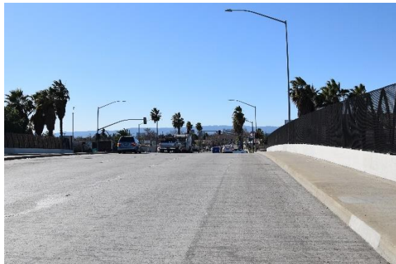
Narrow Sidewalks on Freeway Overpasses
