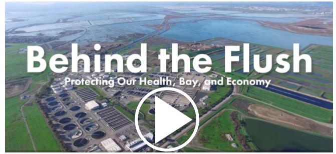
San José-Santa Clara Regional Wastewater Facility
