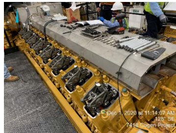
Cogeneration engine during commissioning.
