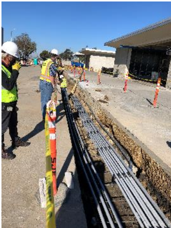
Installation of duct bank conduits for power connection from Headworks 2.
