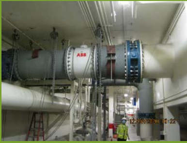
Installation of the nitrification B-side influent flowmeter.
