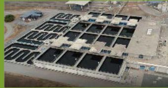
Aerial view of the current filtration area.
