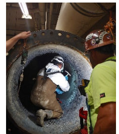
Assessing the condition of a 54-inch pipe.
