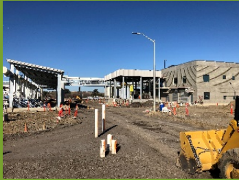
Preparing pavement to the new Sludge Screening Building.
