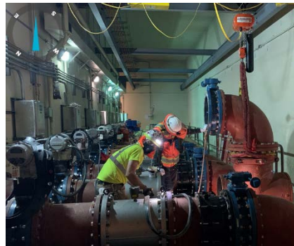
Contractors in the return activated sludge gallery.
