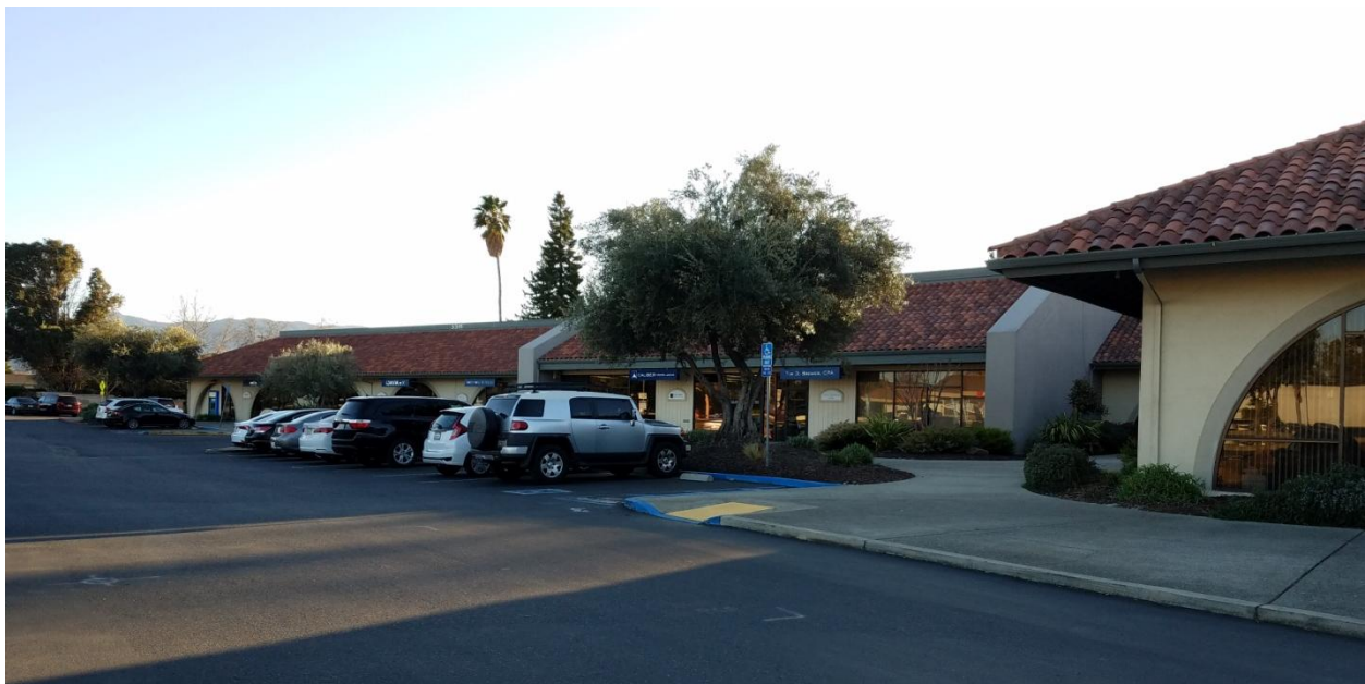
Figure 1. The property is developed with a commercial complex. Nearly all existing structures, landscaping, and hardscape will be demolished to construct a new assisted living facility.
