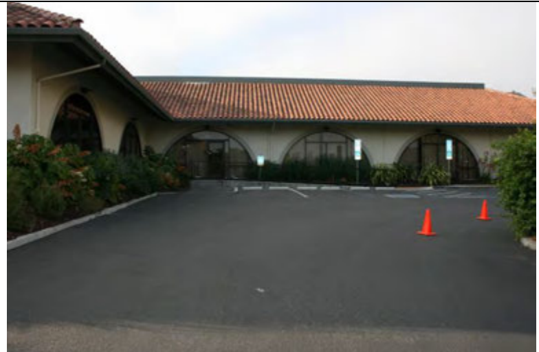
North elevation of on-site building looking South
