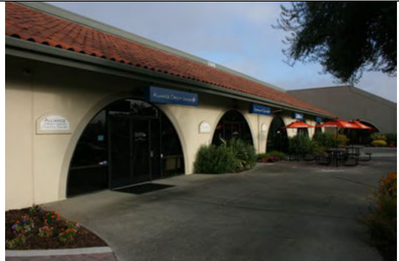
East elevation of on-site building looking North
