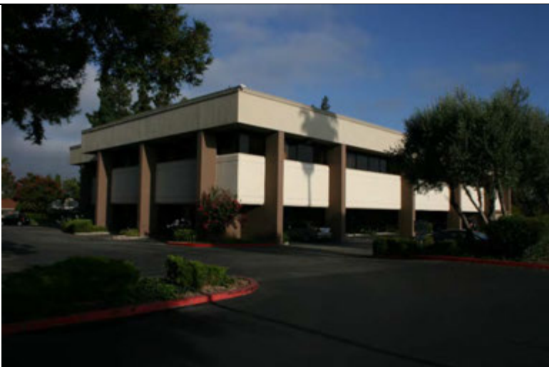
View toward West adjoining properties
