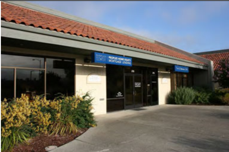
Typical tenant space exterior
