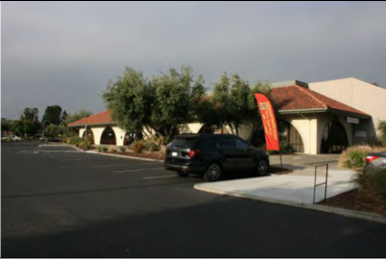
East elevation of on-site building looking Southwest
