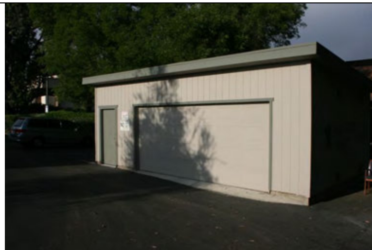
On-site office storage garage
