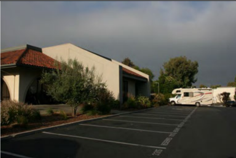
North elevation of on-site building looking West-southwest
