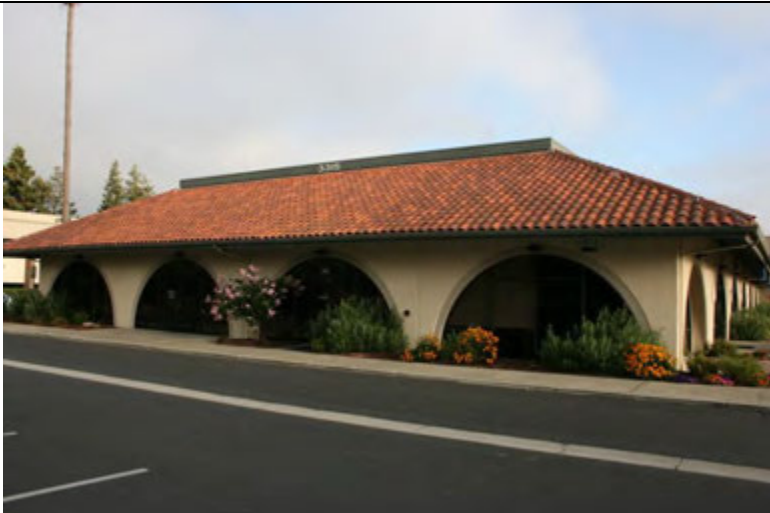
South elevation of on-site building looking North
