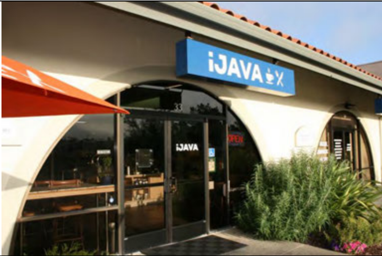
Typical tenant space exterior
