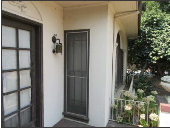
Figure 11. 971 Meridian Avenue Home, Entry Courtyard
