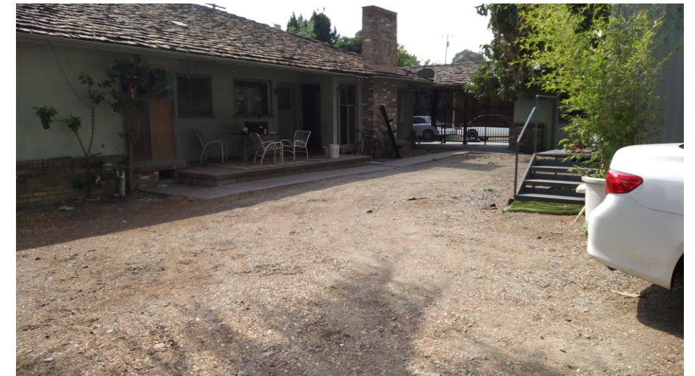
6) Parcel -015 (961 Meridian Avenue), view looking south at rear of existing residence, office-type trailer at right of photograph.
