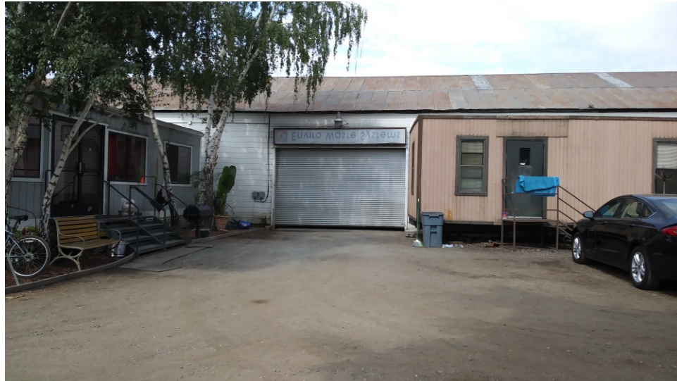
7) Parcel -049 (961A Meridian Avenue), view looking west at southern portion of building front of warehouse building. Current operator has installed two office trailers in front of building
