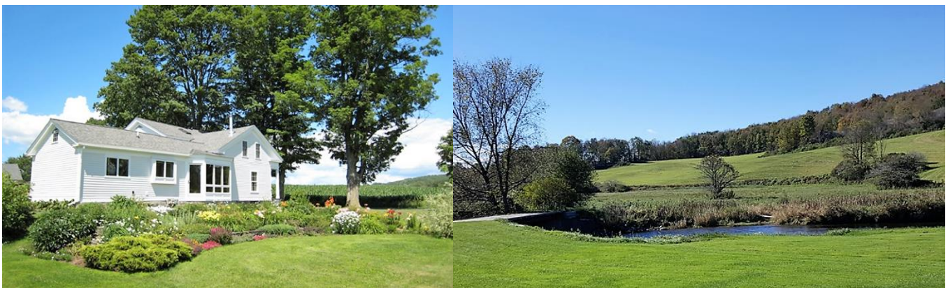
Figure 29: Peter Darby's home that was built in 1830 was retrofitted to be zero emissions and all-electric, including a water source heat pump that uses well water as the heat source, and discharges the water into the adjacent creek. 74
