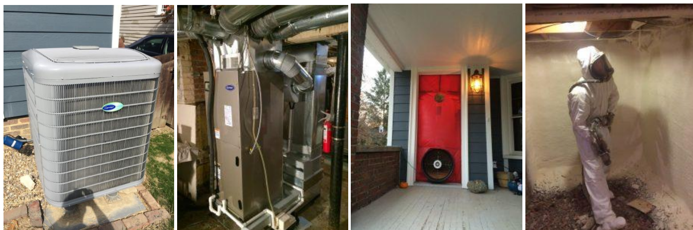
Figure 15: A few images from Energy Smart Ohio’s retrofit project 1918 House of the Future in Cleveland Heights. Left to right: Carrier Greenspeed heat pump, air handler in the basement, blower door test, and insulating the basement.
