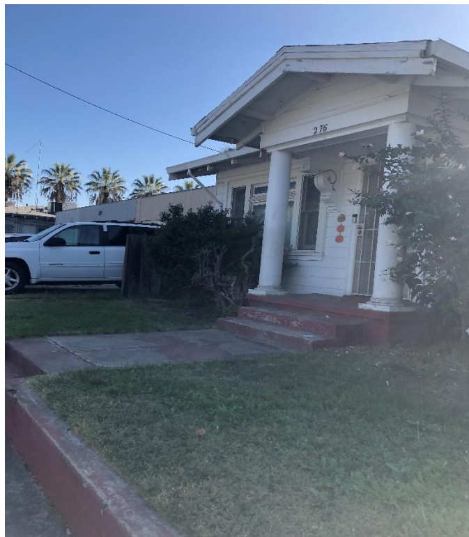
Photograph 8: View of residential building at 276 Woz Way
