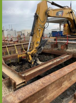
Excavation for the installation of the 96-inch pipe
