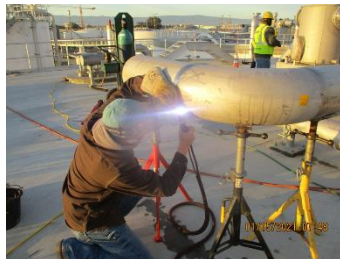
Contractor welding a digester gas line on top of Digester 7.
