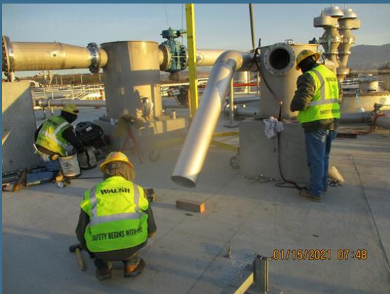
Construction workers observing COVID safety protocols
