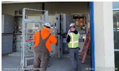
Contractors at the new Tertiary Blower Building electrical room.
