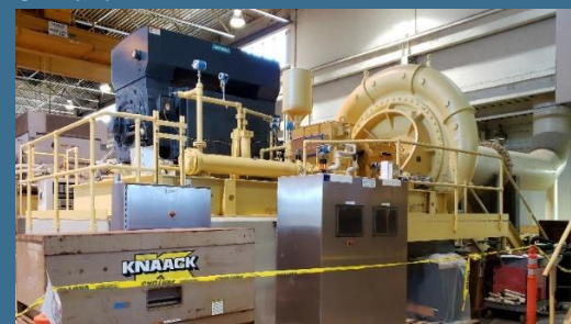
PAB #2 completed and ready for testing
