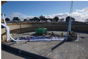
Contractors installing CIPP lining for the RAS B7 pipeline.
