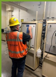
Contractor performing a test on a turbidity meter.
