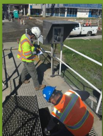
Contractors testing new flow meters.
