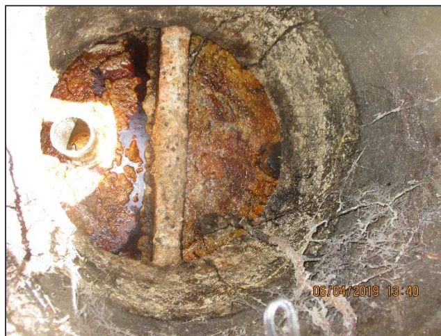
FIGURE 25. INSPECTING A COMMERCIAL GREASE INTERCEPTOR
