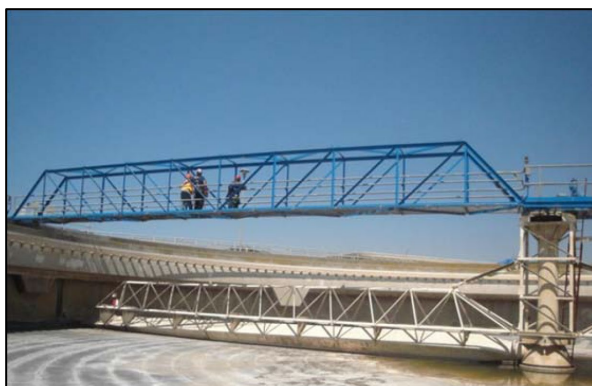
FIGURE 28 WORKER ON A CLARIFIER "TOW-BRO" ARM
