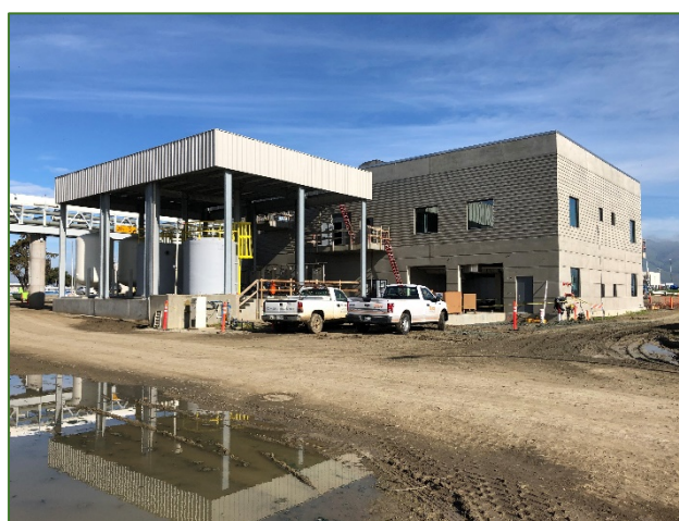
FIGURE 24 NEW SLUDGE SCREENING BUILDING NEARING COMPLETION
