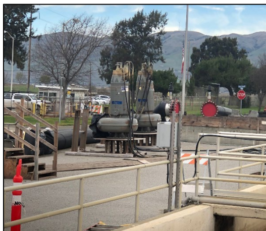
FIGURE 22 TWO OF THE PUMPS UTILIZED IN THE TEMPORARY PIPING SYSTEM THAT WAS USED IN 2018 AND WILL BE USED AGAIN FOR THE SES REHABILITATION PROJECT.
