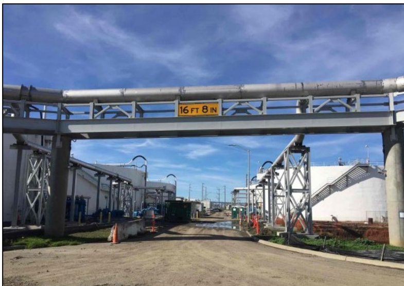
FIGURE 26 NEW PERMANENT ABOVE-GROUND PIPING RACKS: “THE MONORAIL” AT THE REMOTE DIGESTERS
