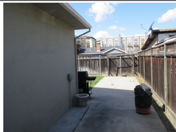
Photo 9: Walkway located at 383 South Baywood Avenue.
