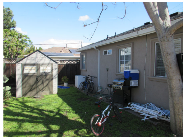
Photo 3: View of the backyard located at 375 South Baywood Avenue.
