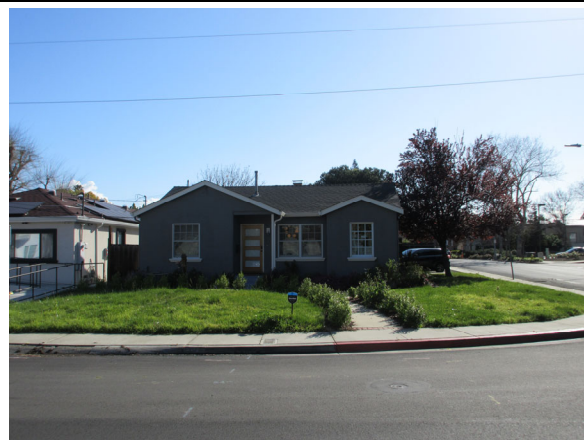
Photo 22: View of 383 South Redwood Avenue.
