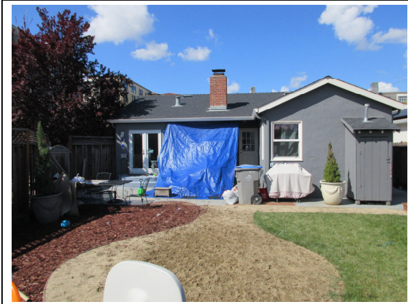
Photo 25: View of the home located at 383 South Redwood Avenue.
