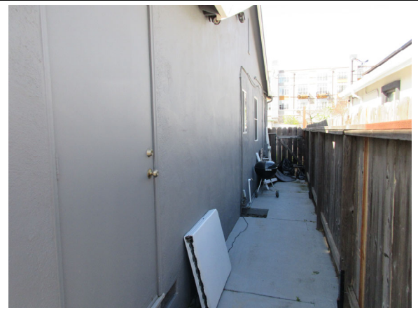
Photo 266: View of a walkway located on 383 South Redwood Avenue.
