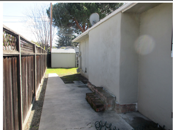
Photo 10: Walkway located at 383 South Baywood Avenue.
