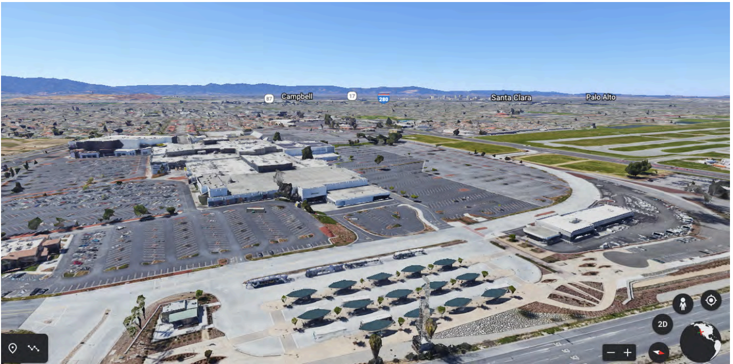
Aerial view Eastridge Station (existing view looking west towards Mall)
