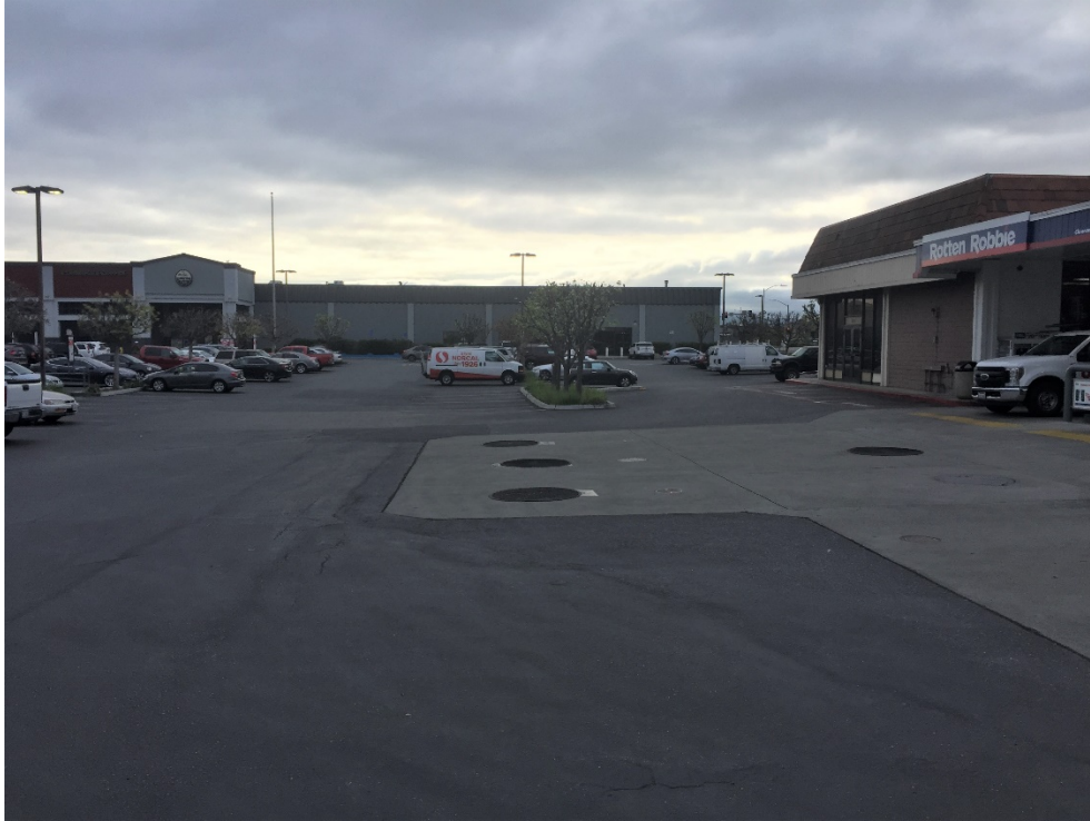
1 – View of the northern portion of the Site, where the concrete pad and access holes for the existing USTs are located. The main shopping center building is visible to the east of the Site in the background. Looking east from the northwest portion of the Site.
