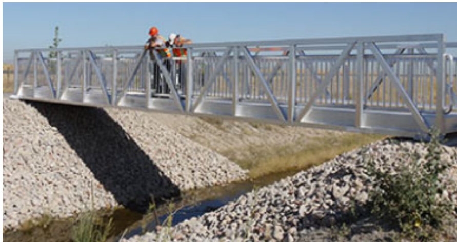
Photo 2: Pre-Fabricated Aluminum Bridge
