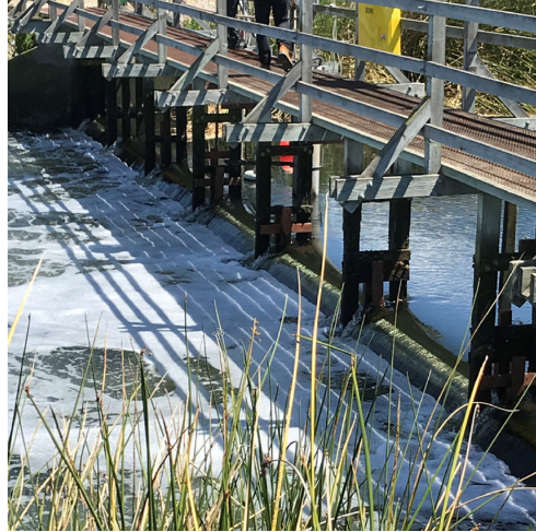
Photo 1: Existing Outfall Bridge and Weir
