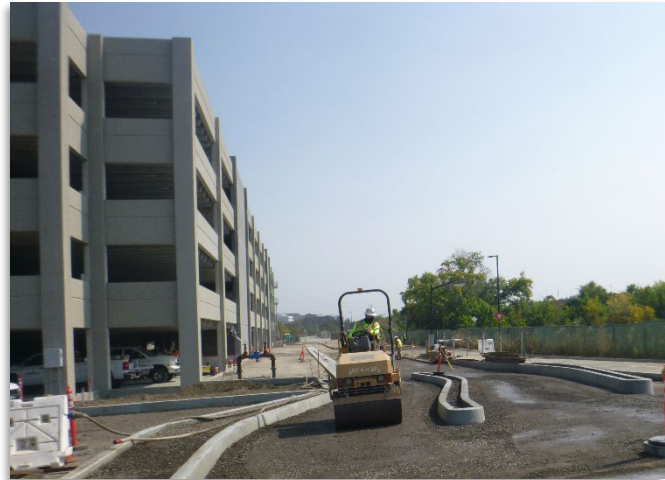
Economy Lot 1 Parking Garage under construction
