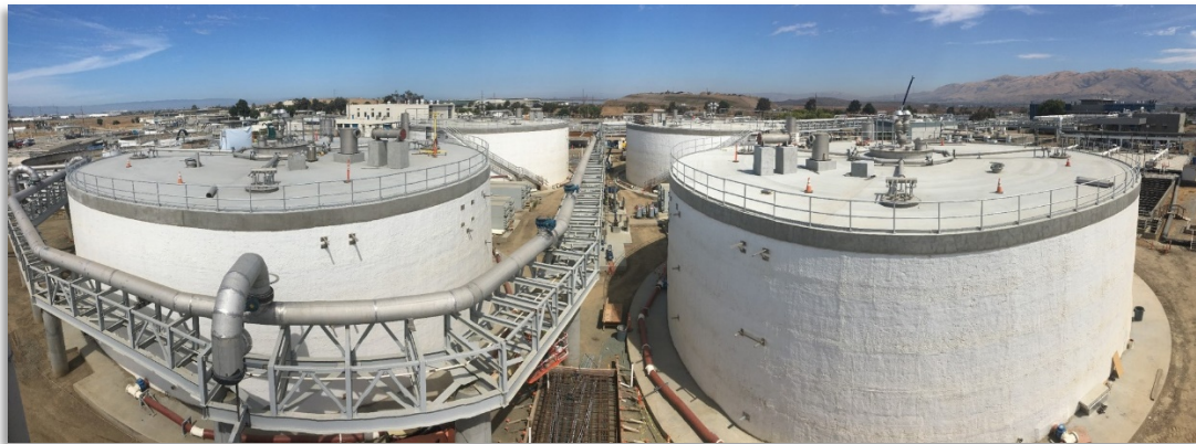
Upgraded Digester Facilities
