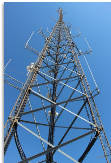
Transmitter Antennae at Coyote Peak
