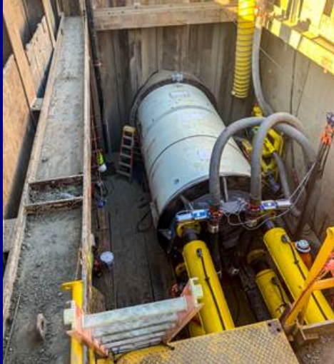
Fourth Street 84-in Interceptor Phase VI-A Project (tunneling operation)
