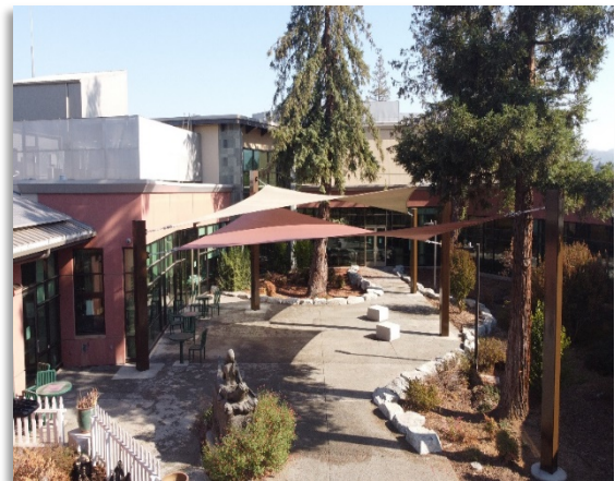
Almaden Community Center Structure
