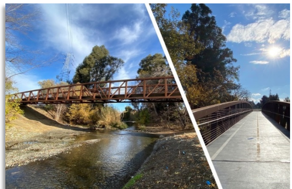
Three Creeks Trail Pedestrian Bridge
