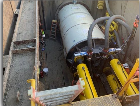
Fourth Street 84-inch Interceptor Phase VI-A
