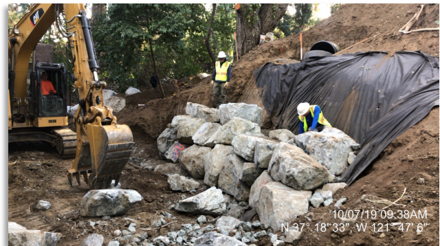
An outfall being rehabilitated on Thompson Creek
