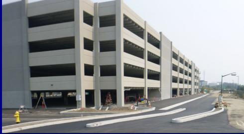
Economy Lot 1 Parking Garage at the Airport
