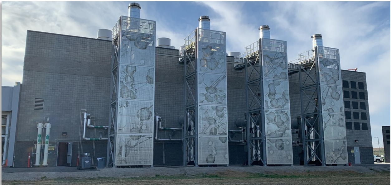
New Cogeneration Engine Building
