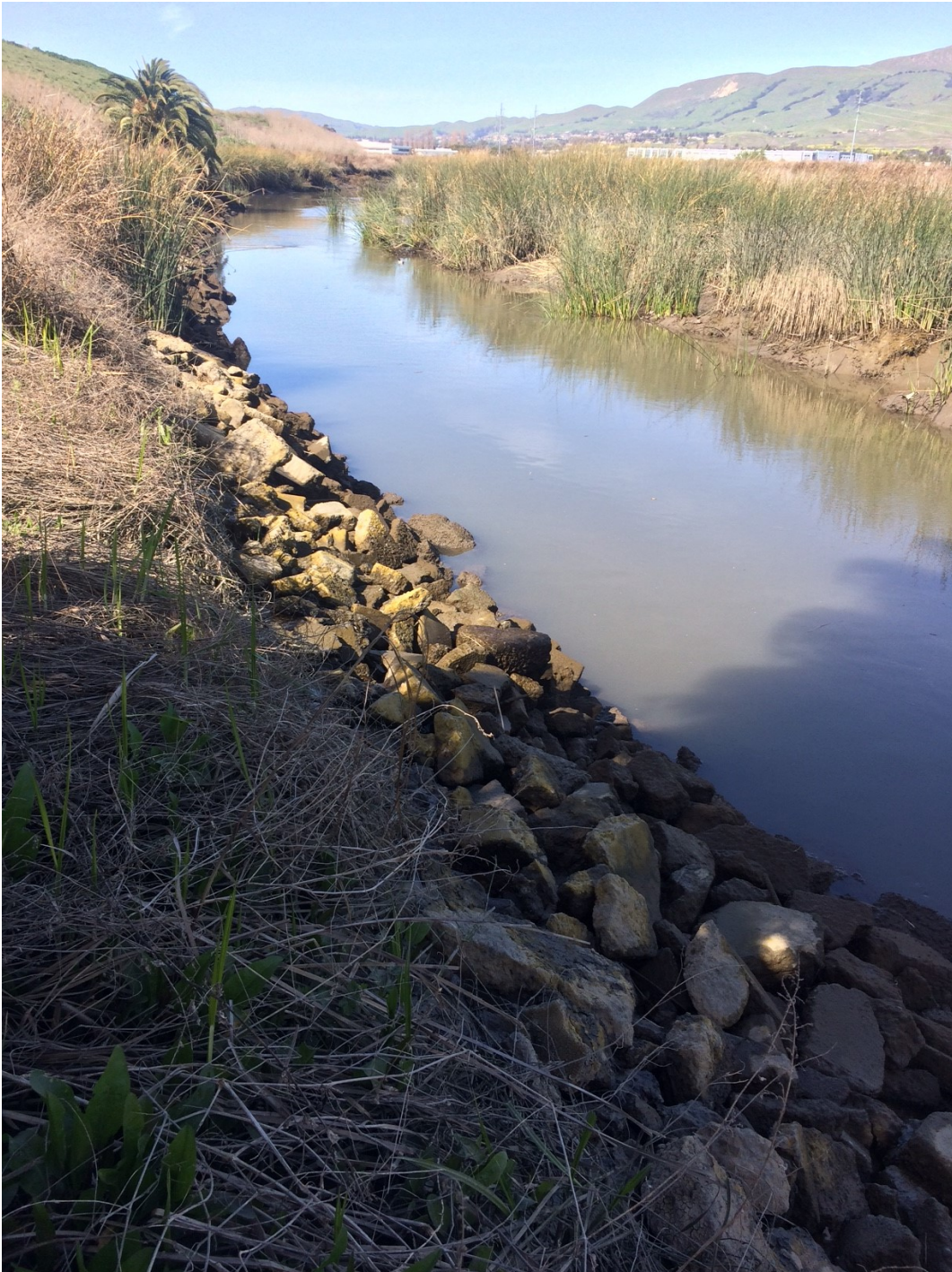
Photo 3: Existing revetment along Coyote Creek immediately downstream of Project site
