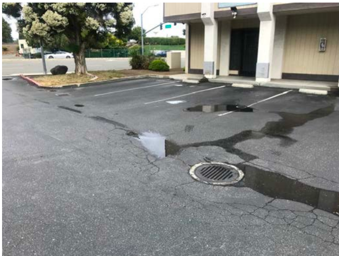
9. View of an area drain and pooled water.
