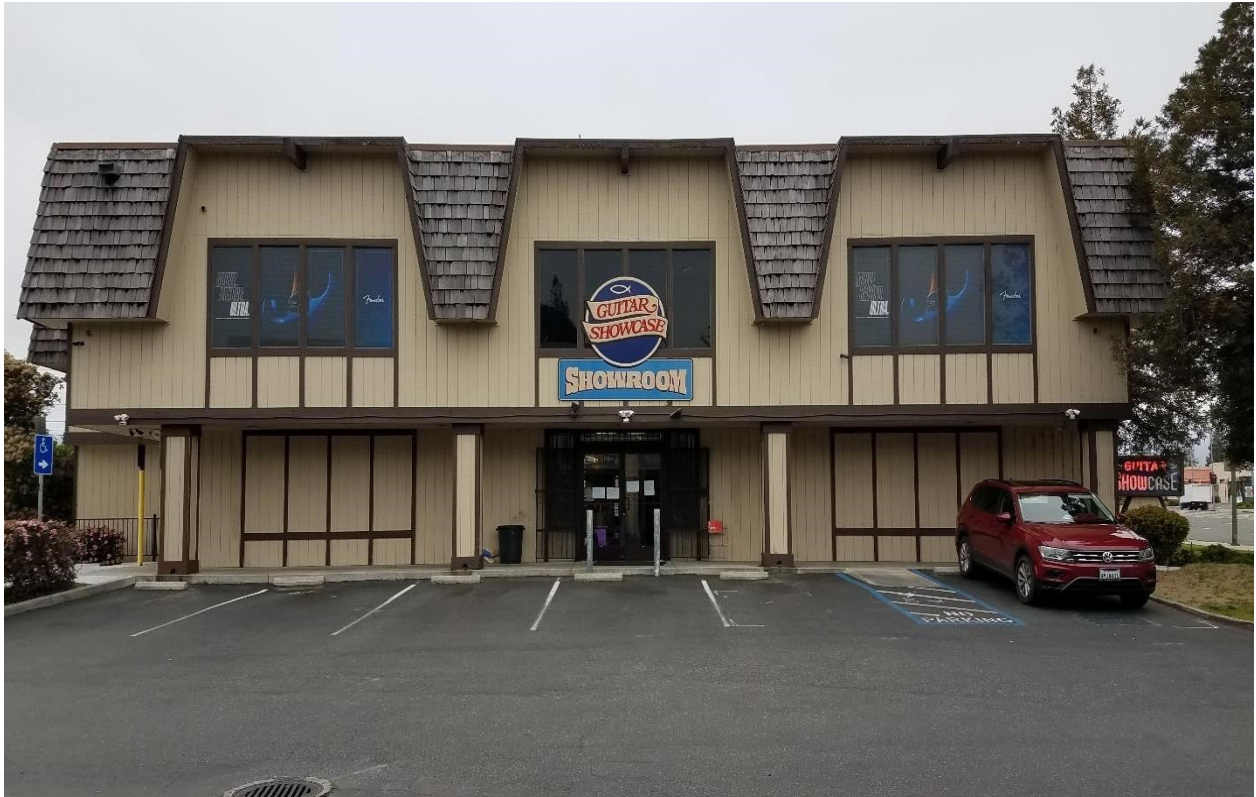
Photo 1— Northern Façade, View Looking South
