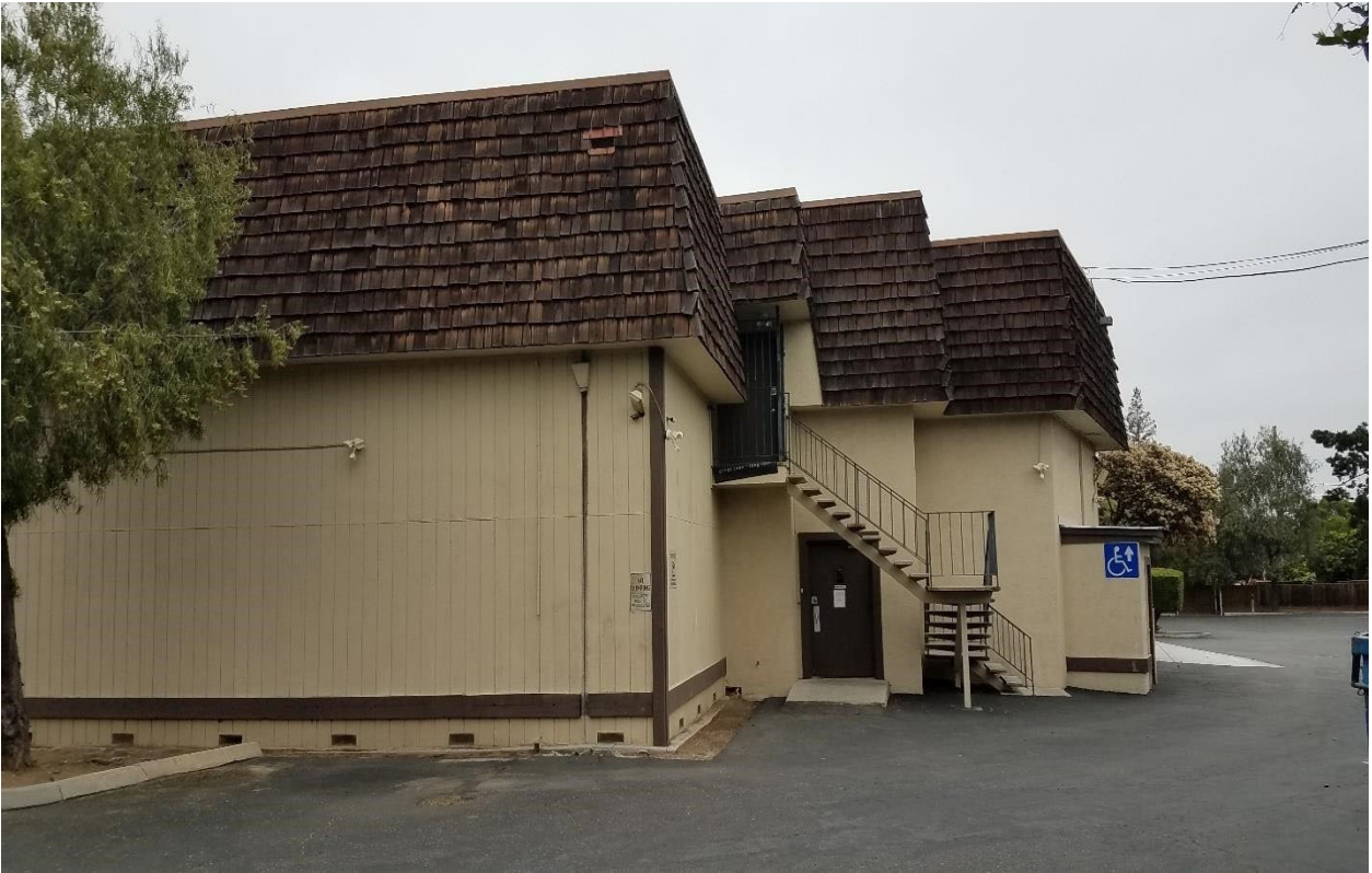
Photo 4— East Elevation, View Looking West
