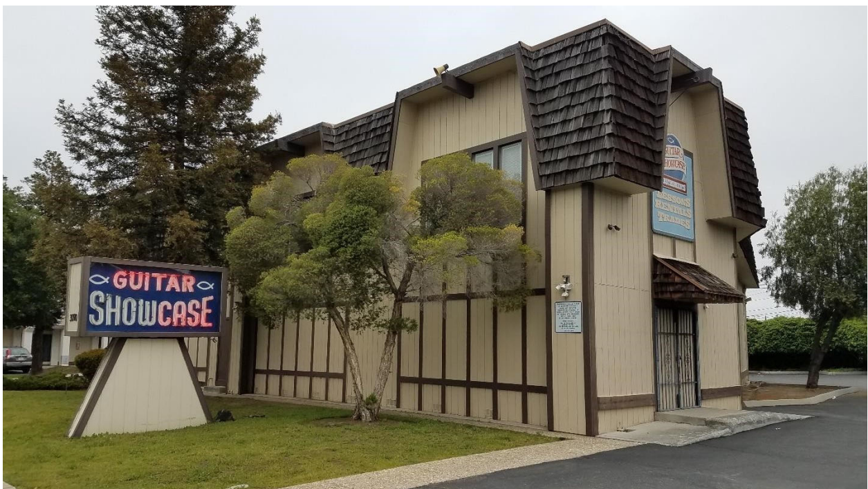
Figure 4b— Site Photographs
