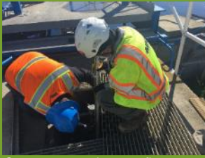
Contractors testing new flow meters.
