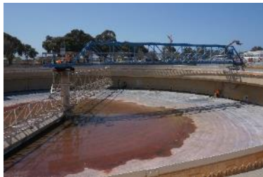
Contractors inside an empty clarifier.
