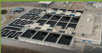
Aerial view of the current filtration area.
