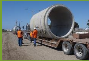
Contractors next to a section of the 96-inch pipe.
