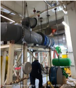
Valve installation at the Tertiary Blower Building basement.
