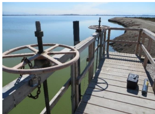
Pond A18 condition on September 28, 2016.
