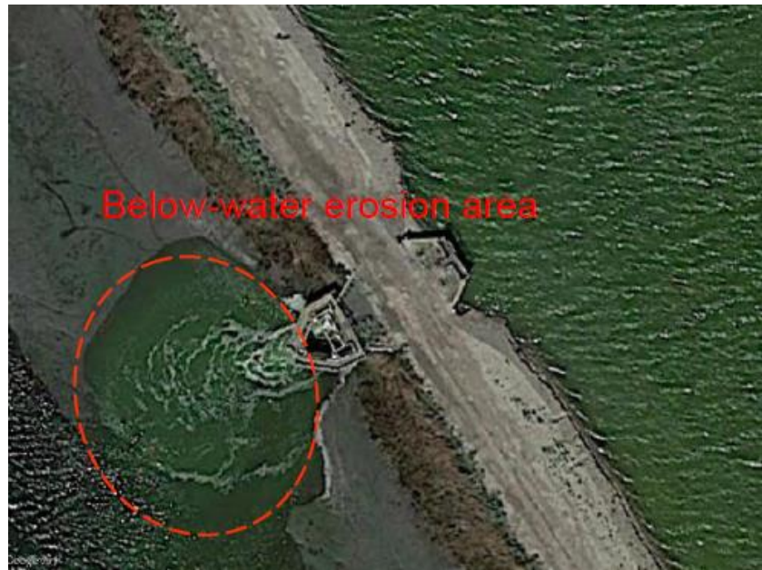
Google Earth satellite imagery details the erosion on the outboard side of the southern hydraulic structure.
