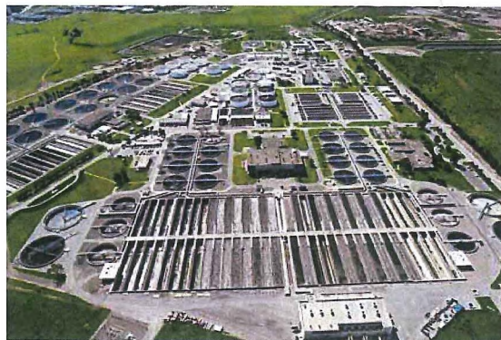
Aerial View of the Water Pollution Control Plant
