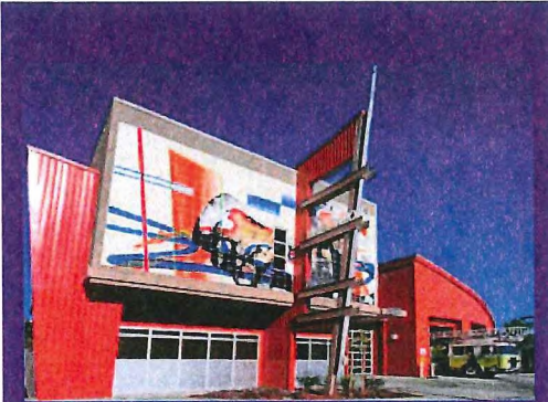
Fire Station 2 - Rebuild
