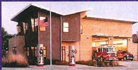
Fire Station 19 (Piedmont)
