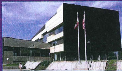
South San José Police Substation
