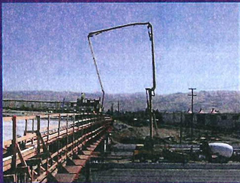
Route 101/Tully Road Interchange Reconstruction
