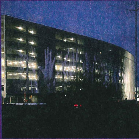
Airport Rental Car Garage
