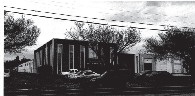
VIEW FROM ROGERS AVENUE - EXISTING CONDITIONS
