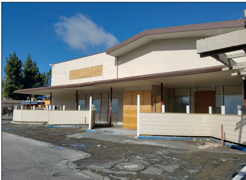
Photograph 2. Rear elevation camera facing northwest, February 12, 2021.
