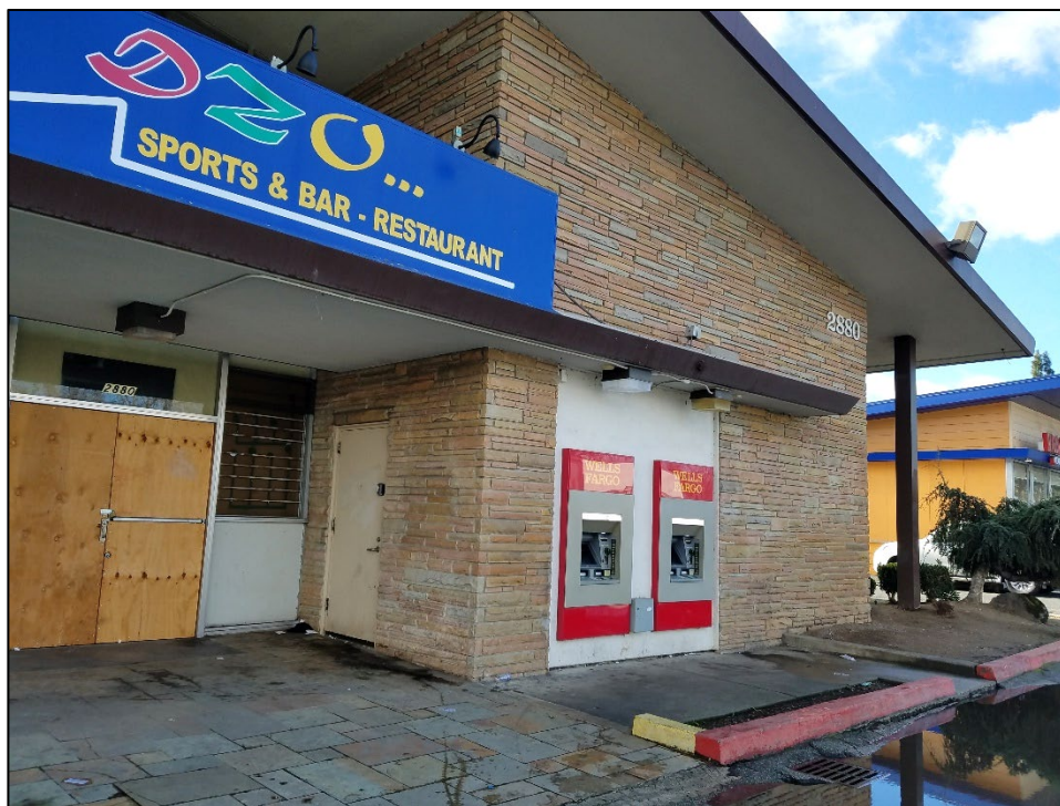
Photograph 5. Main entrance (left) and single metal door in façade bay with ATM machines, February 12, 2021.
